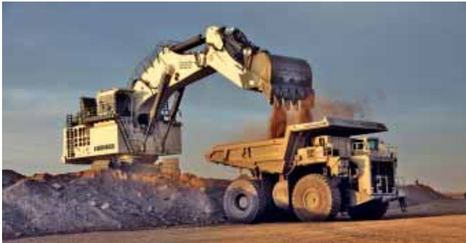
One of two Liebherr 996 excavators at Ovoot Tolgoi
